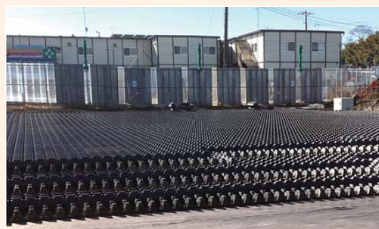
Work to lay AQUAROAD
